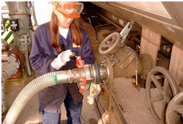
Bottom loading of Ethylene Oxide
